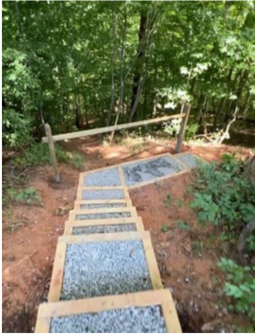
New steps are installed at Fisher Farm Park in Ridgeway, VA.
